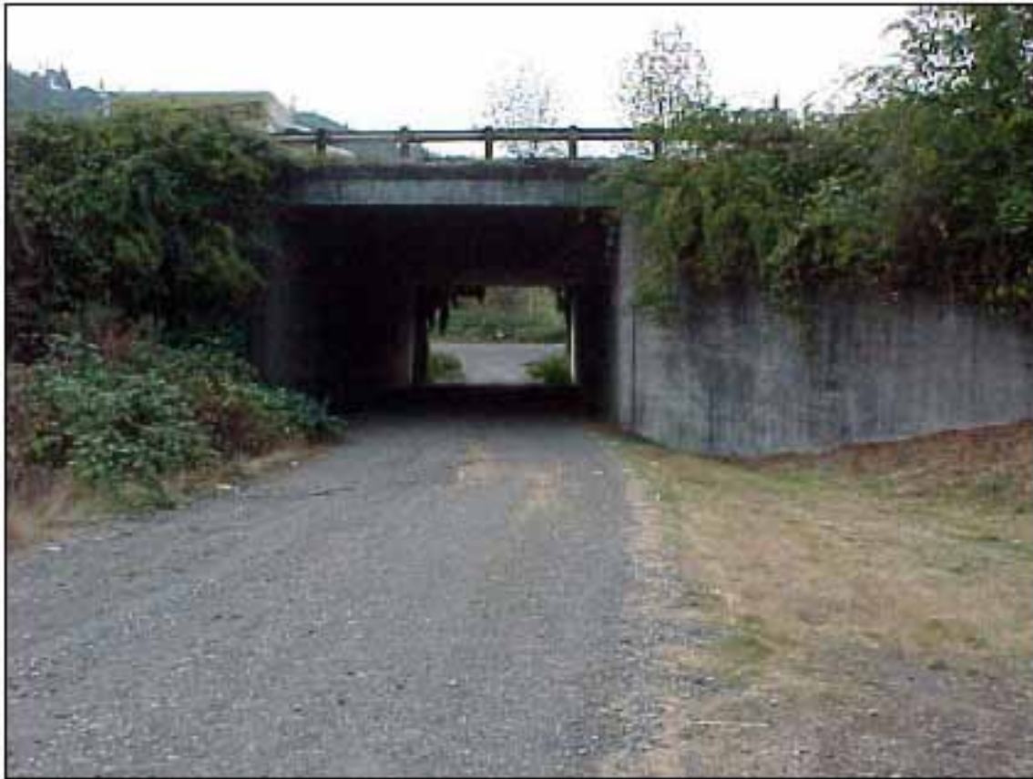
Bridge 08870 - Hwy 1 over Hwy 225 Connector (McVay Access):
