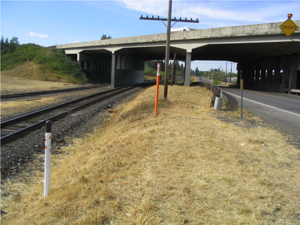
Bridge 06836A - Hwy 1 over Franklin Blvd & UPRR (Goshen):
