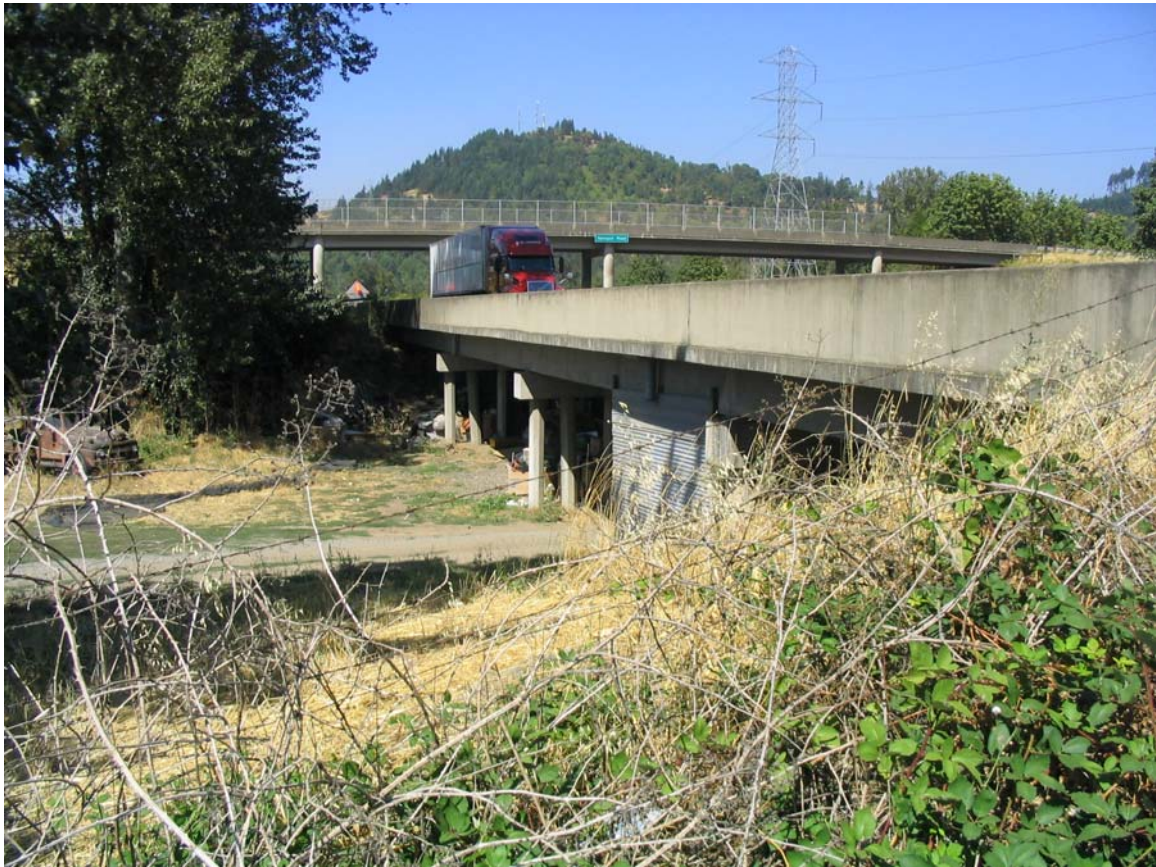
Bridge 08178S - McKenzie Oflow, Hwy 1 SB at MP 196.69:
