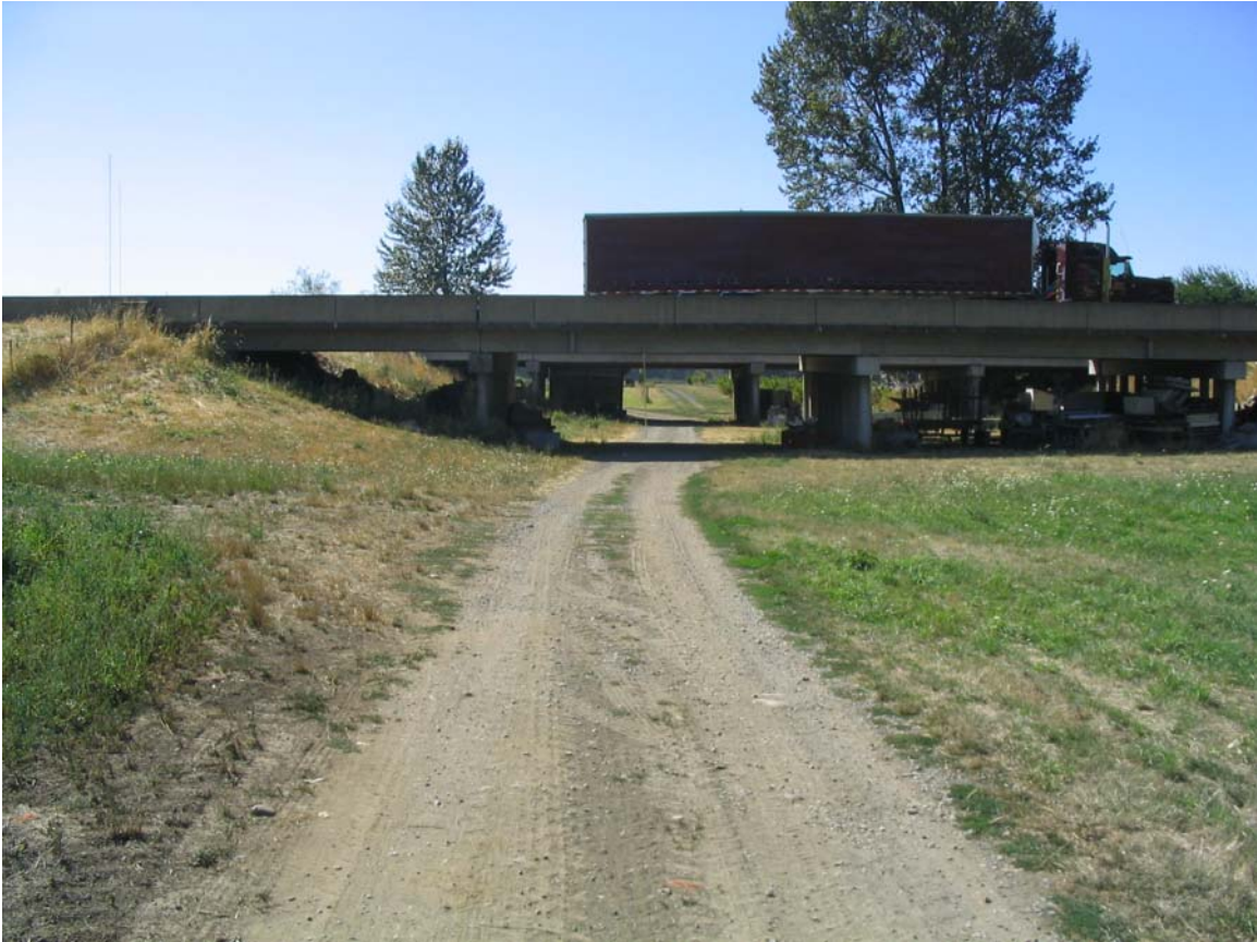
Bridge 08178N - McKenzie Oflow, Hwy 1 NB at MP 196.69:
